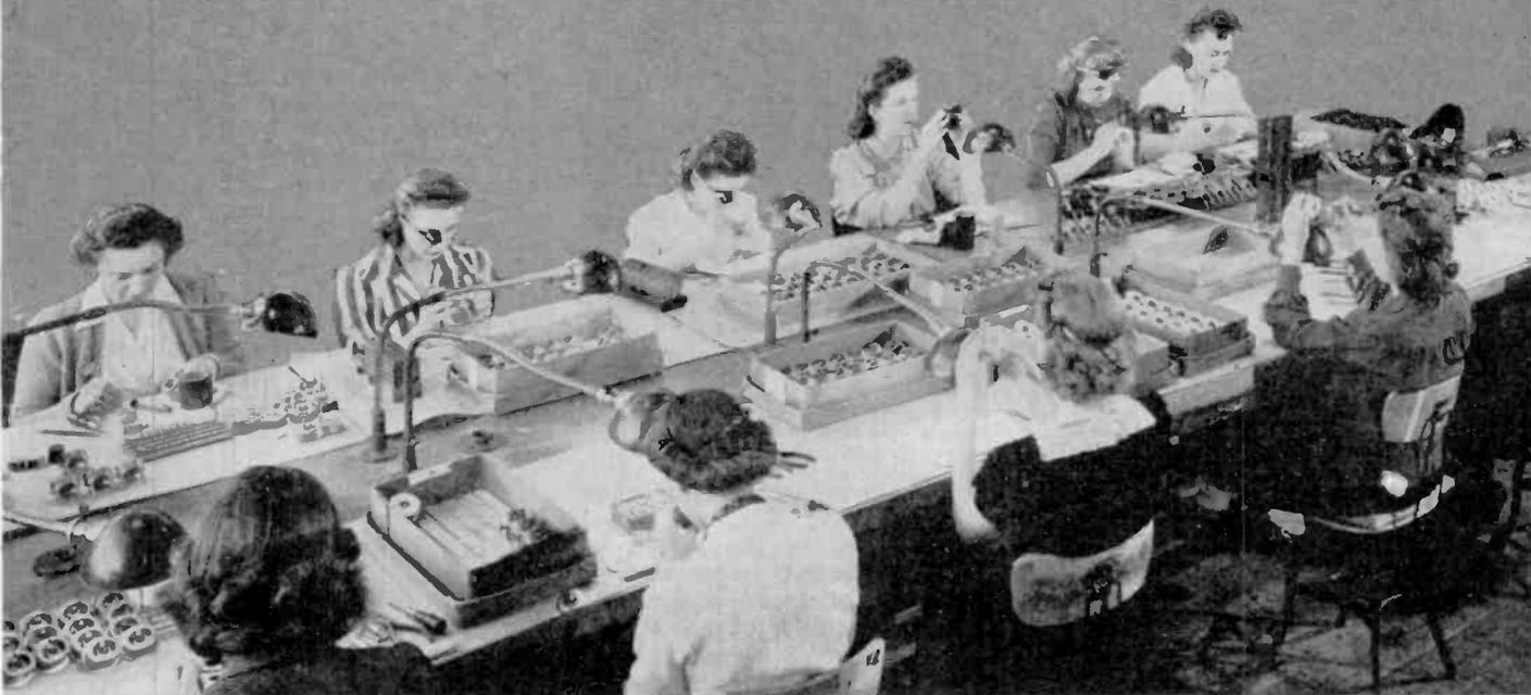
**6. JEWELER'S EYE LOOP** facilitates delicate assembly and adjustment of meter movements in Western Electric's Chicago plant. Eye loops cost from fifty cents to a dollar or two per operator
