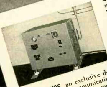
**AUTO-DRY-AIRE**, an exclusive development of Communication Products, is a completely automatic device for maintaining coaxial transmission lines at pre-set pressures of moisture-free air. It will function for indefinite periods at the rate of 1000 cubic inches per minute. It is independent of critical gases and heavy cylinders.
