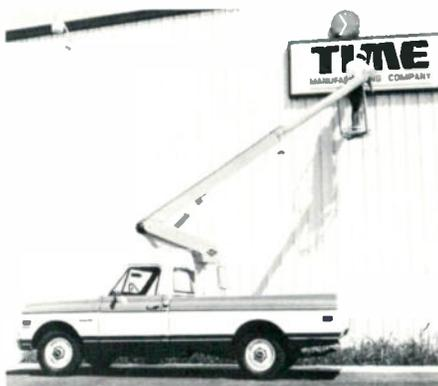
Use of an aluminum upper boom with a simplified drive and power system have resulted in a total unit weight of 1200 pounds.
