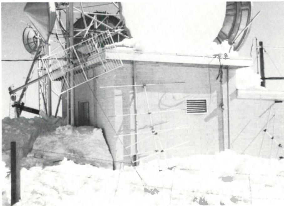
*The storm on Pinal Peak near Globe, Arizona left the cable system's antennas strewn around the head-end site. The channel 12 antenna appears to be vertically polarized!*
