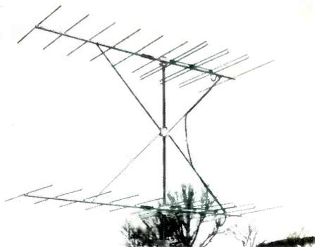
Stacking of the ruggedized antennas is facilitated because of the use of coaxial terminations. Tuned lines terminating in coaxial connectors provide a perfect match with full weather protection. Bracing of the antennas is by means of sturdy aluminum rods fastened to antenna and mast by special brackets. Twisting of the antenna "boom" which can cause flutter is eliminated by use of rectangular tubing to which the welded elements are sturdily attached.
