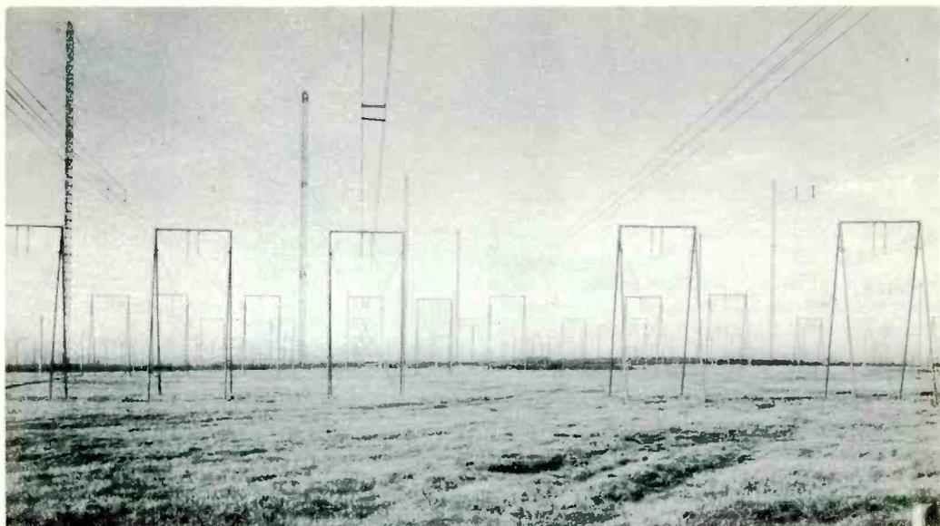
Antennas—antennas everywhere... as far as the eye can see. A "portion" of the BBC General Overseas Service Antenna System, seemingly stretching to the horizon. The four wire feeder systems are supported by the smaller towers. The larger towers support the actual antennas, "Sterba Curtains" mostly.
