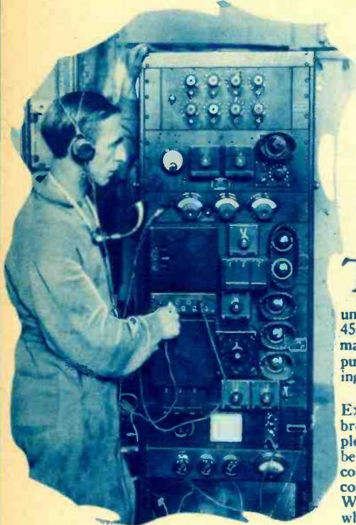
Front view of the speech input panel. Note the multiplicity of meters, tubes, coils, pilot light, switches, jacks, plugs and relays. Surely a complicated system, but it is only one part in the endless detail of an efficient up-to-date broadcast station.
