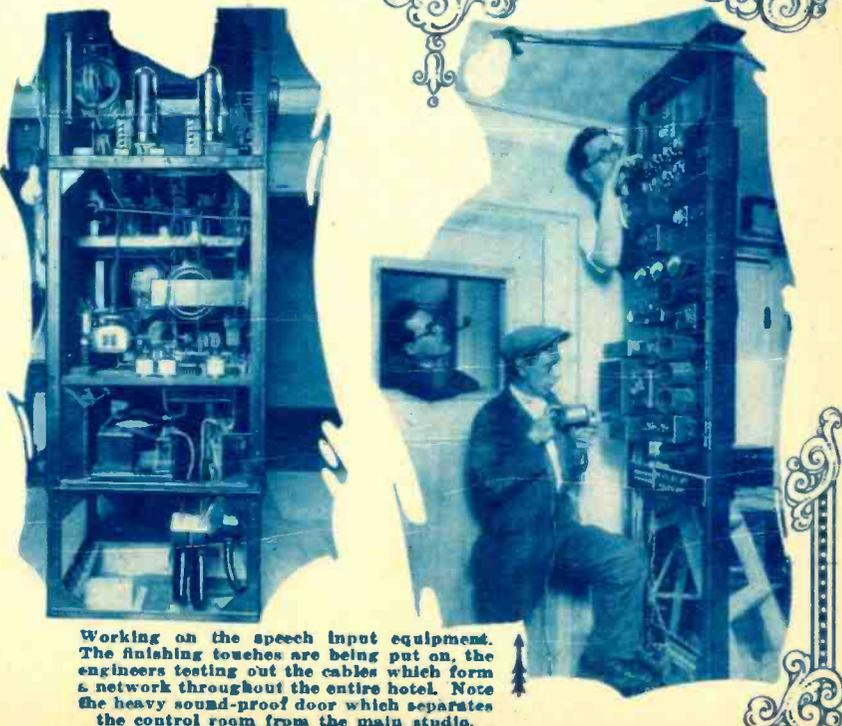
Working on the speech input equipment. The finishing touches are being put on, the engineers testing out the cables which form a network throughout the entire hotel. Note the heavy sound-proof door which separates the control room from the main studio.
