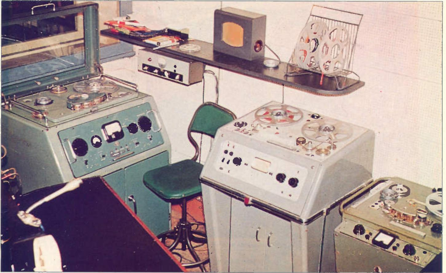
Studio A control room. Left to right: bottom left, STC value mixing desk; EMI BTR2 recorder; WIFOS reverb control unit — under shelf; Philips recorder and EMI TR90 recorder
