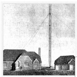
The new transmitter site had to allow for a tall tower, as horizontal aerials in broadcasting were being relegated to history. Vertical towers acting as the radiator take less space and can be heightened to a wavelength that matches the transmitting frequency. The match allows maximum efficiency of output power.
