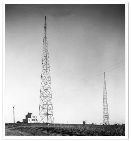
WAAW Towers at 60<sup>th</sup> and Girard Streets. Nearly invisible is the antenna strung between the top of the two towers, it's feed line dropping straight down from the center point to the small building below. (1931) (Courtesy Durham Museum)
