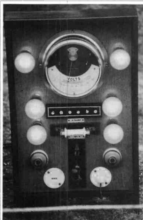
**Fig. 2: A beautifully restored distribution board, originally used to supply low-voltage lighting in country houses.**
