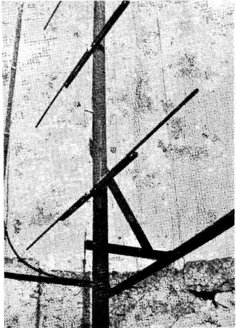
Construction of the 16-element stack at G5TZ/A, with its wire-mesh reflector. The Old Light House, long since abandoned, on St. Catherine's Point — from where G5TZ/A operates on two metres — is a very lonely spot 780 feet a.s.l. An important item in his equipment is a rifle — to keep the wild life under control and possible intruders at bay!
