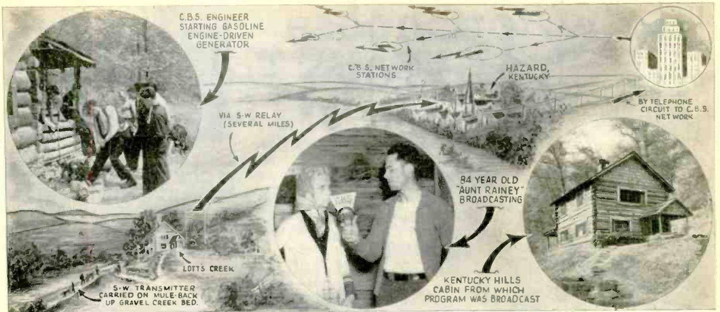
Above—Several interesting angles of a recent short-wave broadcast pick-up which originated at Lott's Creek, Kentucky. As no electric light or power lines were available, a gasoline engine and dynamo supplied power for the short-wave transmitter, which served to relay the broadcast to the CBS network.
