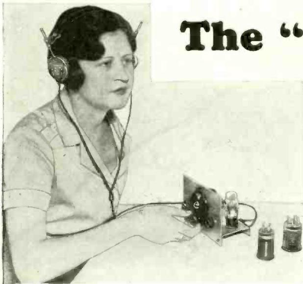
At the first trial of the "19" Twinplex, a battery-operated one-tube receiver, foreign, as well as American stations, rolled in with amazing smoothness.
