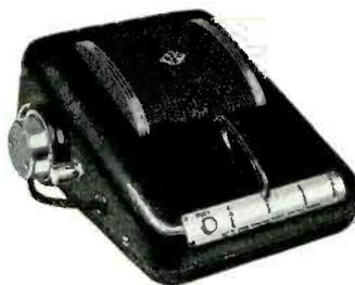
Call-Phone which is equipped with an earphone. Raising the earphone from its rest makes conversation confidential by bringing the other party's voice over the earphone instead of the loudspeaker. Other units in the system include the Standard Call-Phone, which has no earphone, the Switchboard Call-Phone for use by telephone operator in extensive installations, and the Paging Call-Phone which amplifies the call over large areas.
