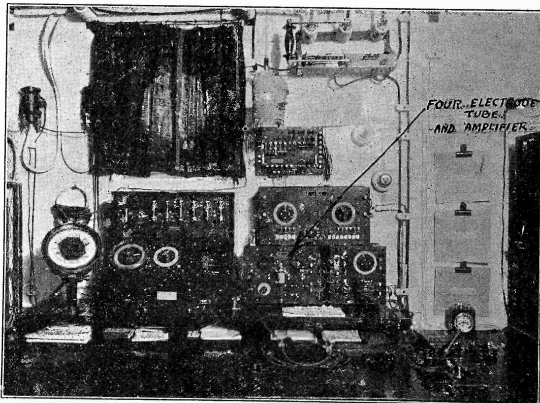
Four-Electrode Tube In Use on Atlantic Liner.
