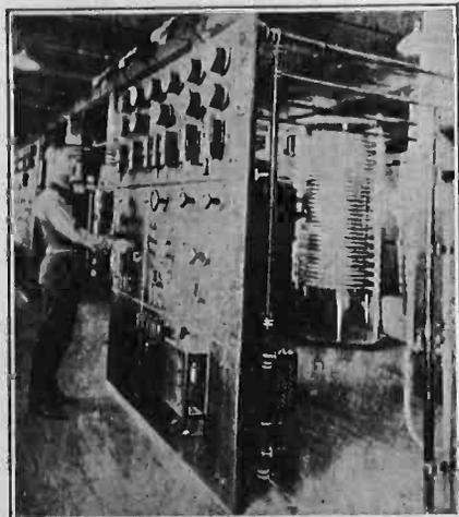
*Control Panel of 80 K.W. Tube Transmitter at San Diego.*
