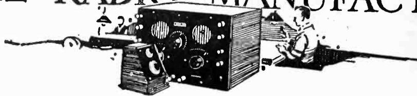
The Metralign SLT variable condenser has plates so designed as to give equal dial spacing or straight line tuning for all stations. The construction is so rugged that constant use will not change
