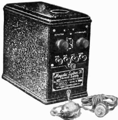
multi-tube sets with power tube in the last stage. It uses a Raytheon tube as a rectifier and has three adjustable resistances controlling the voltage delivered to various tubes.
