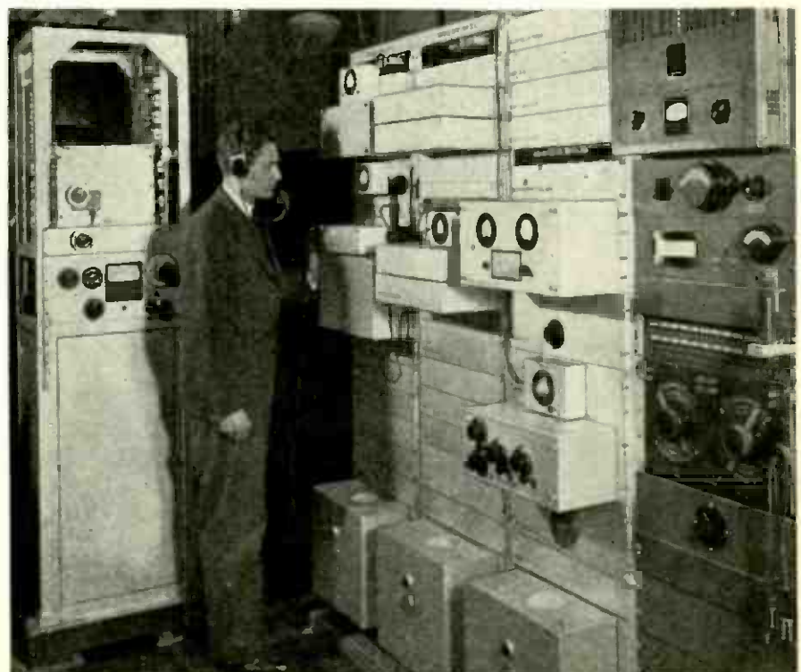
FIG. 9 Modulating terminal equipment at the New York end of the coaxial circuit.
