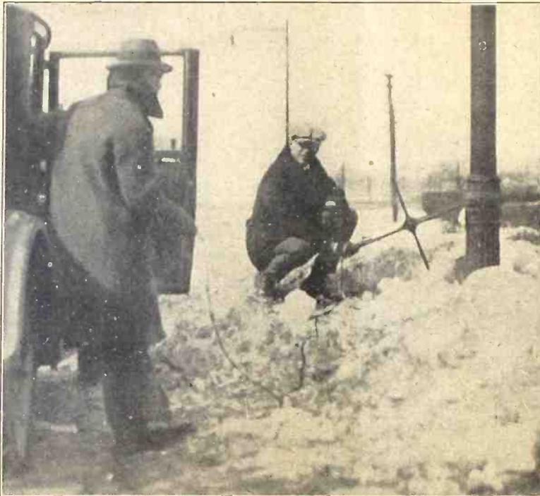
A NOVEL and ingenious method of finding out where broken cables are present, with the use of a radio receiver, has been put into use by some large power companies in the eastern portion of the United States. A super-sensitive receiver, employing a loop as the collector of energy, is used to detect the stray noises. (Underwood & Underwood)
