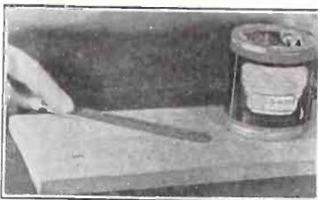
PUTTY may be used as a filler to plug up a hole in a wooden baseboard.
