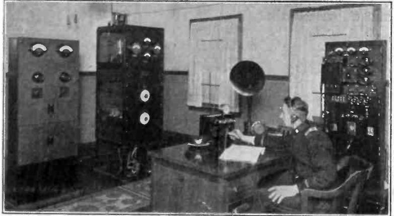
Operating room of Station WCBD, Zion, Ill. On the extreme right is the Western Electric speech amplifying control board. In front of the operator on the opposite side of the room are the transmitter control panel and the transmitter tuning panel.
