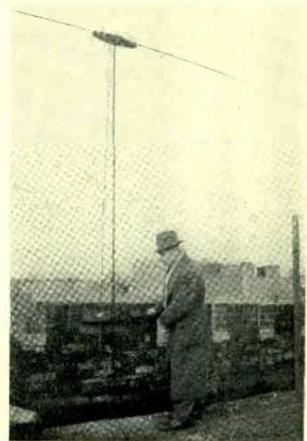
Fig. 3. A good antenna installation. Mounted in the clear and securely fastened by expansion bolts. Twisted-pair feeder is used
