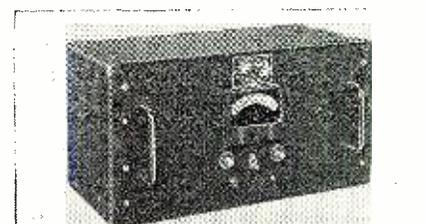
inch voltmeter, an "on-off" switch, pilot light, and screwdriver adjustments for output voltage and sensitivity.
