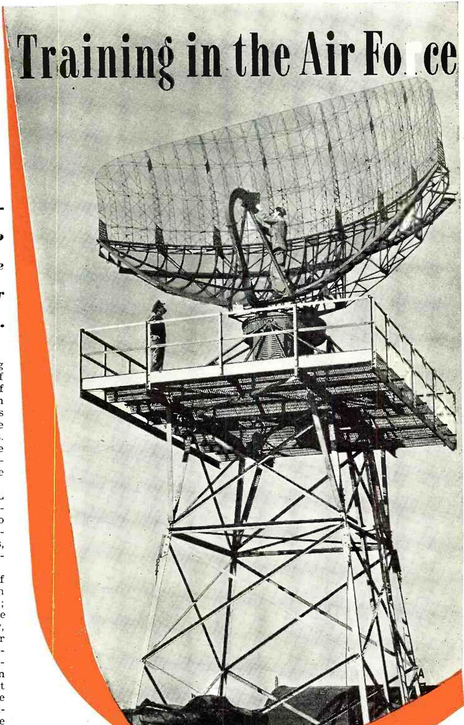
Student adjusting a feedline on an aircraft warning radar.
