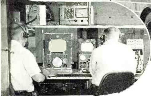
television control room, with wide panels of glass installed on three sides to permit broad vision from inside the control room. Television cameras are set up on a table stretching across the room, with three revolving seats provided for WTMJ-TV engineers. Above the table is a shelf for sound equipment, while down in front there is room for the cables to be run to the scene of the pictures.
