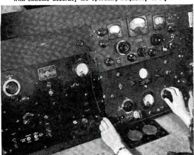
An array of electronic equipment which is used to determine with extreme accuracy the operating frequency of crystals.
