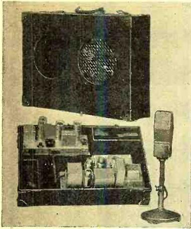
pensation switch. Provisions have been made to supply polarizing voltages for a carbon type microphone. Single or double phonograph turntable units mounted in individual carrying cases are available as auxiliary equipment to this sound reproducing system. Sound engineers, radio dealers and servicemen should find more than ordinary interest in this public address system as a profitable item for rental or sale, for installation in auditoriums, dance halls, etc.
