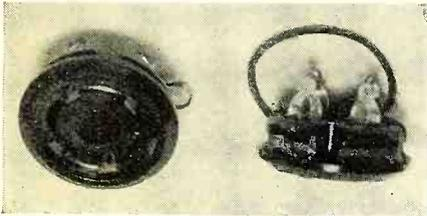
sible short connecting leads and also makes possible the interchange of various type sockets in the same mounting holes. This type of socket design permits tube shields to be mounted underneath the socket without employing chassis fasteners or rivets. These sockets are available in different models to take all the vacuum tubes now in active use.
