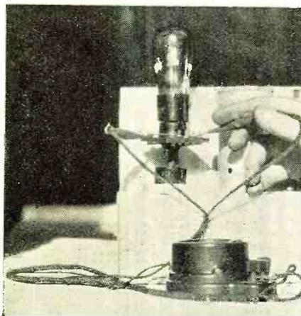
milliammeter in series with the plate circuit. The terminals were marked with white ink; two of which have two certain letters corresponding to the elements in the different tubes as shown in the picture.
