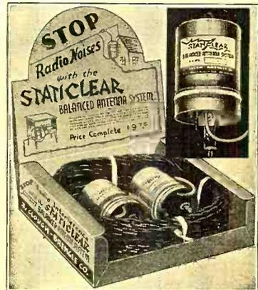
mission line, two radio-frequency transformers to match the antenna and receiver input impedances to the balanced transmission line, and complete mounting hardware. This system is designed for use with either broadcast or short-wave antennas.
