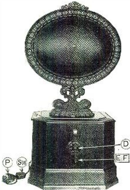
One tuning dial (D) controls the wavelength of this receiver. P is the volume control and E is an additional sensitivity control, Sw turns the set on and off.
