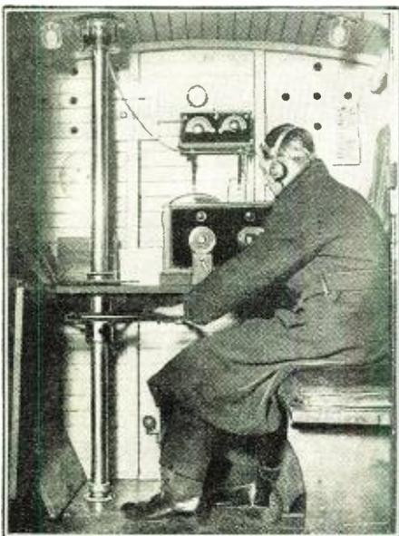
THE motor equipment here illustrated was built for the use of the British post office, which has jurisdiction over radio, as well as all telephone and telegraph service in the United Kingdom; and is now being utilized to detect oscillating sets, which are prohibited by law.
