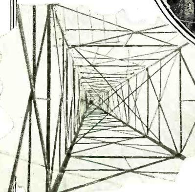
This steel spider web is what you would see on looking up the interior of one of WRNY's masts, which are 127 feet high; they are of the latest type of construction and braced to withstand high winds, because of their exposed position on top of the Palisades.
