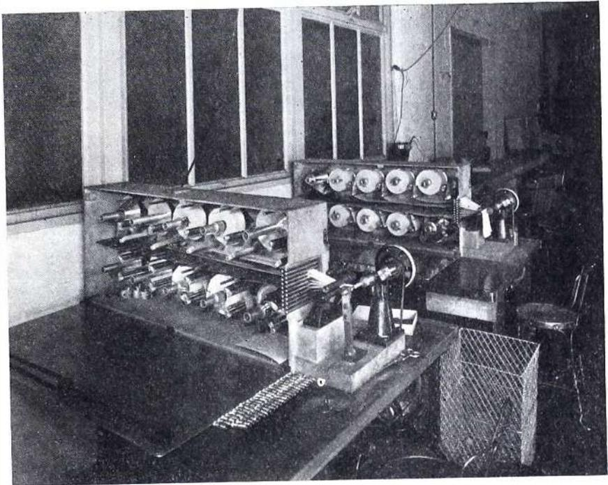
Two of the condenser winding machines. The rolls of paper and tin foil can be seen inside the metal casings
