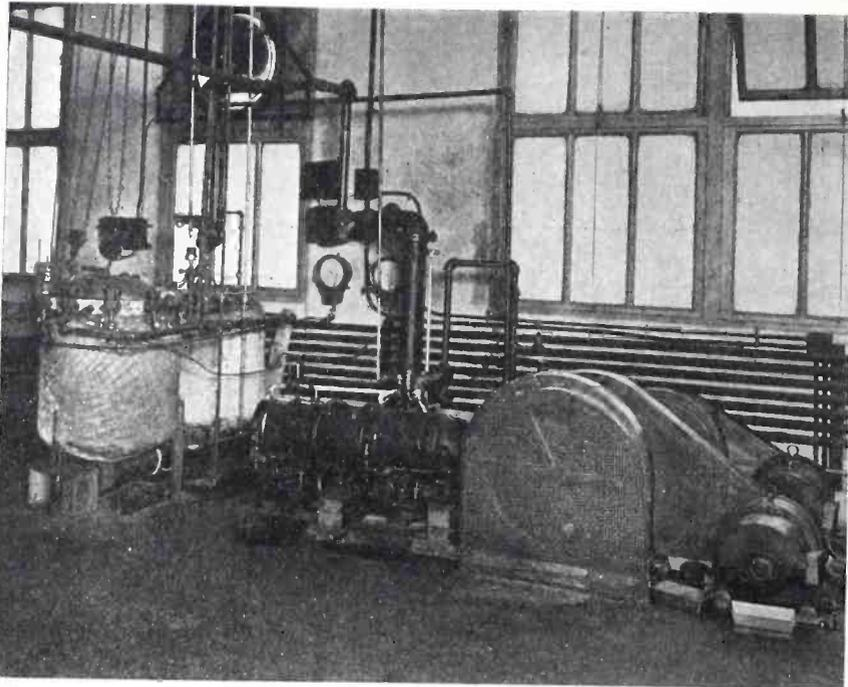
Two of the condenser impregnating tanks and, to the right, the immense electric driven vacuum pumps
