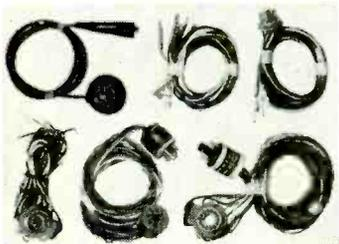
**COLOR SERVICE HARNESSSES AND ADAPTORS.** Line consists of CRT extensions, anode extensions, convergence deflection-magnet extensions and adaptors. With the CR-506, a 48-in. socket extension cable for all 21-, 23- and 25-in. color tubes, the chassis can be removed from set, leaving CRT connected.—I. E. H. Mfg. Co.
