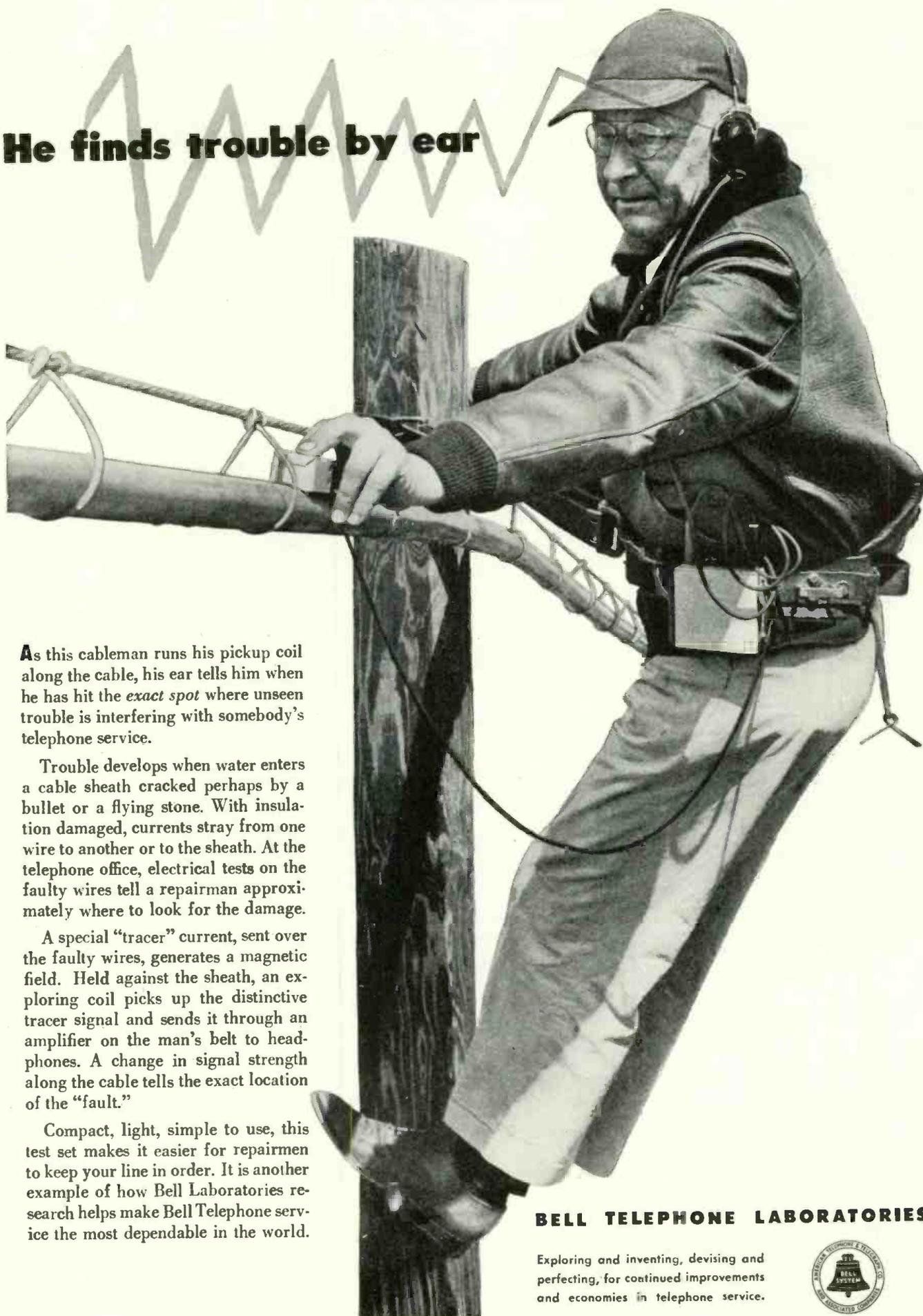
As this cableman runs his pickup coil along the cable, his ear tells him when he has hit the *exact spot* where unseen trouble is interfering with somebody's telephone service.
