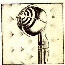
CARDIOID CRYSTAL-LABYRINTH MICROPHONE The Shure "Uniplex" 730-A is a diaphragm-type unit with uni-directional cardioid characteristics (obtained through the addition of an acoustical labyrinth).
