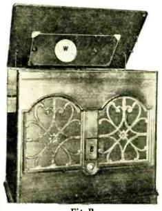
Fig. B The mirror in the console lid reflects the image on the target of a "kinescope" set below it.
