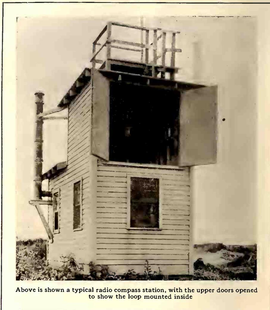
Above is shown a typical radio compass station, with the upper doors opened to show the loop mounted inside
