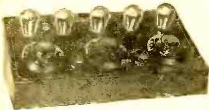
This is known as the "Marwol Baby Grand," and comes equipped for storage battery use, but may be changed to operate on dry cell tubes.
