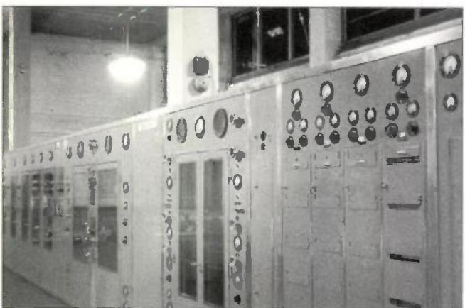
Sender 10 was withdrawn in 1969 when two Marconi H1200 30kW single sideband transmitters (SSB1 and 2) were commissioned, with three rhombic aerials. These transmitters were later converted for independent sideband operation, i.e. two sidebands carrying different programmes, SSB1 and 2 were withdrawn in 1985, when overseas relay stations received their programme feeds by satellite.
