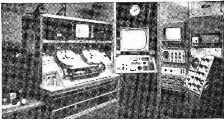
*An R.C.A. TR22 video tape recorder with BBC equipment bays for monitoring at various points. Sound and vision faders, a stabilising amplifier, vidicon caption camera for identification and telephone control panels are all included. BBC photo.*
