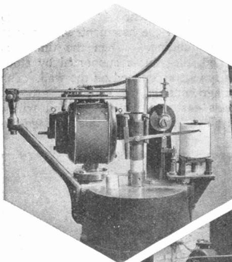
IMPACT MACHINE TO TEST CEMENTING VALUE
