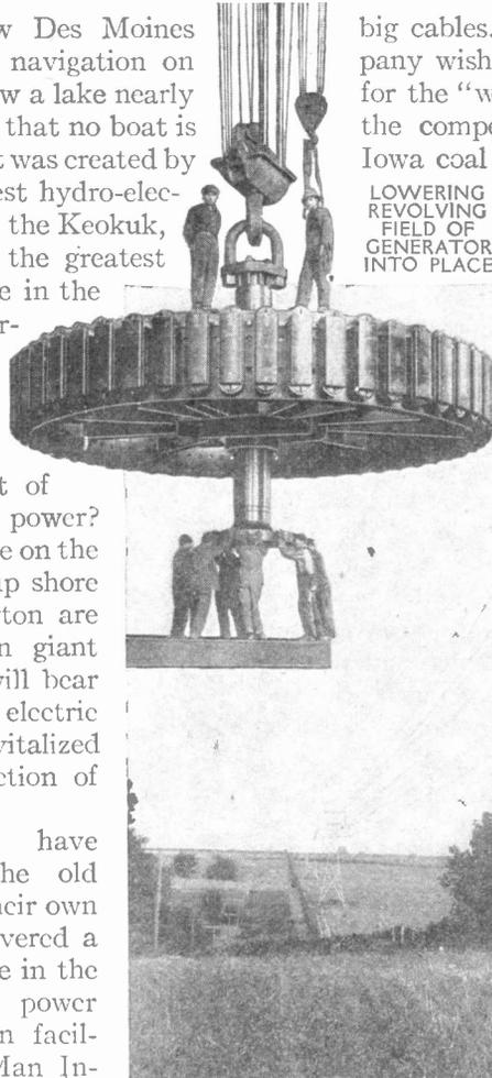
LOWERING REVOLVING FIELD OF GENERATOR INTO PLACE
