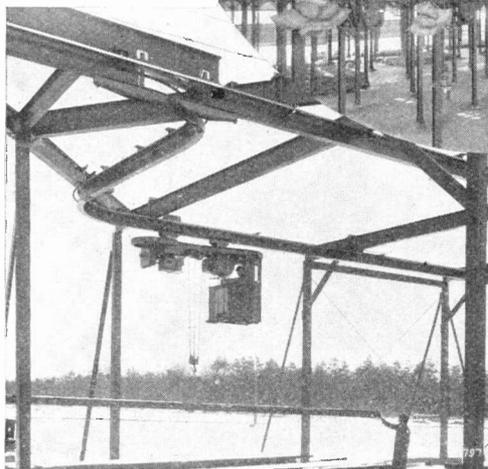
FLEXIBLE METHOD OF SWITCHING IN MONORAIL SYSTEM
