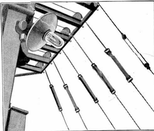
ARRANGEMENT FOR RAISING AND LOWERING ANTENNA WIRES
