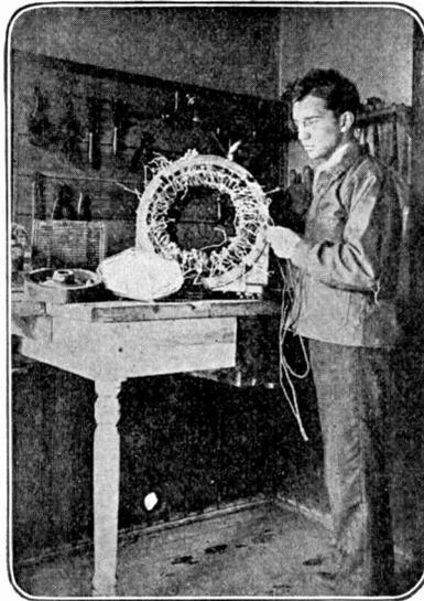
WINDING AN ARMATURE
