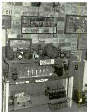
*A 50-watt amateur "phone" station of the early 1920's. Note the carbon hand microphone hanging from table top at right, and the array of chemical rectifier jars on the center shelf.*
