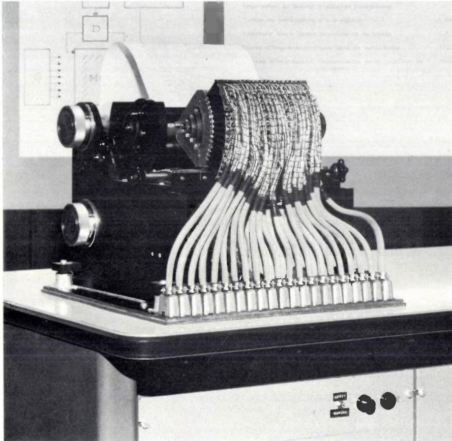
Fig. 16. Experimental model of the line printer, for printing lines of 63 characters at a speed of 2400 lines a minute.
