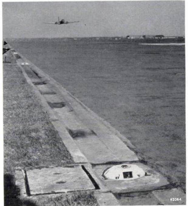
*Fig. 21.* Flush runway light on runway 05/23 at Schiphol. The light is housed in a cast-iron case, and contains two systems of the type shown in *fig. 20*, mounted back to back, and an omni-directional top light. To make the housing watertight, a rubber ring is inserted in a circular groove in the cover, close to the securing bolts. The lower part of the housing accommodates three supply transformers.
