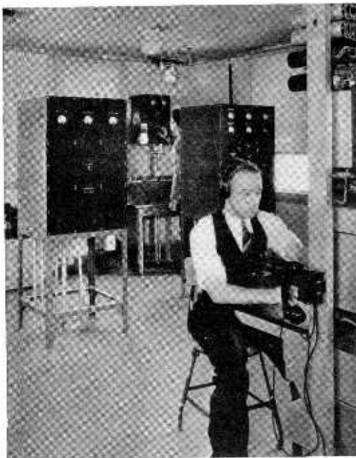
Interior of transmitting and receiving station at Green Harbor, Mass., where calls pass to and from fishing boats off the Massachusetts coast. Photo courtesy Western Electric Company.
