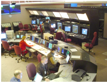
FAA ARTCC Control Room (Courtesy FAA)
