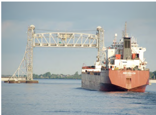
Birchglen approaching St. Louis Bridge on the Seaway.
