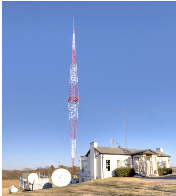
Amore traditional shot of the WSM transmission facility (Courtesy: Bryan Turner)
