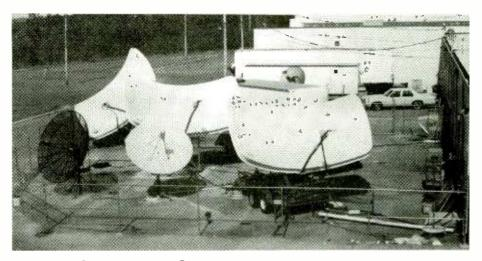
Dish farm at Shop At Home. Signals to three satellites are uplinked from their backyard via the three rectangular parabolic antennas. The two in front are beamed at F4, the one in the back is beamed at G1. The three small dishes are down-link only used to monitor the transmissions. Note the trailer under the foremost dish making it portable.
