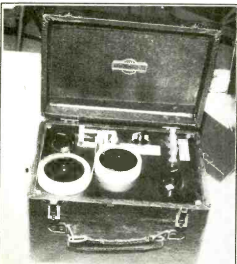
An early code tape reader. The paper tape had punched holes which activated a key. The principle is similar to a player piano roll. Circa 1910.
