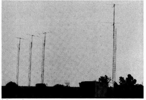
A Transtrack meteor burst remote base station in rural Missouri uses Yagi antennas on the three towers at the left to receive and dual turnstile antennas on the tower at the right to transmit a potent 2,000-watt signal on 43.92 MHz.
