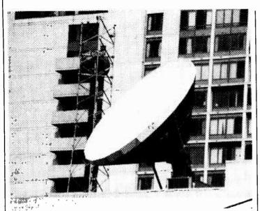
The Satellite News Gathering System (SNG) operates on the Ku band -- 14.0 to 14.5 GHz uplink, 11.7 to 12.2 GHz downlink.
