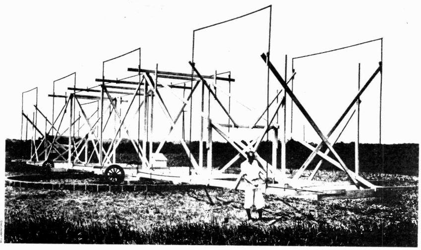
A photograph of Karl Jansky with the rotating antenna (designed to operate near 21 MHz), which he used to discover radio emissions from space. Bell Labs photo.
