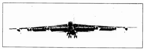
The enormous radar signature of the giant B-52 bomber forced the development of the B-1 bomber which has a radar cross section only 1/100 of that of the older aircraft.
