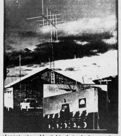
Five-element steerable Qubical Quad. Insert shows Johnson Viking II (100 watts input) transmitter for 26020 kHz.
