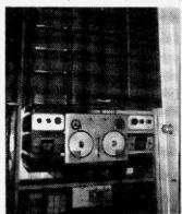
The Dual divercity one (DD-1) 1937-38 25 tubes - audio chosses power supply chasses are located in speaker cabinet which also contains the Jensen 15" coaxiol ≫ speaker. The tuner chassis is on top of the speaker cabinet.
